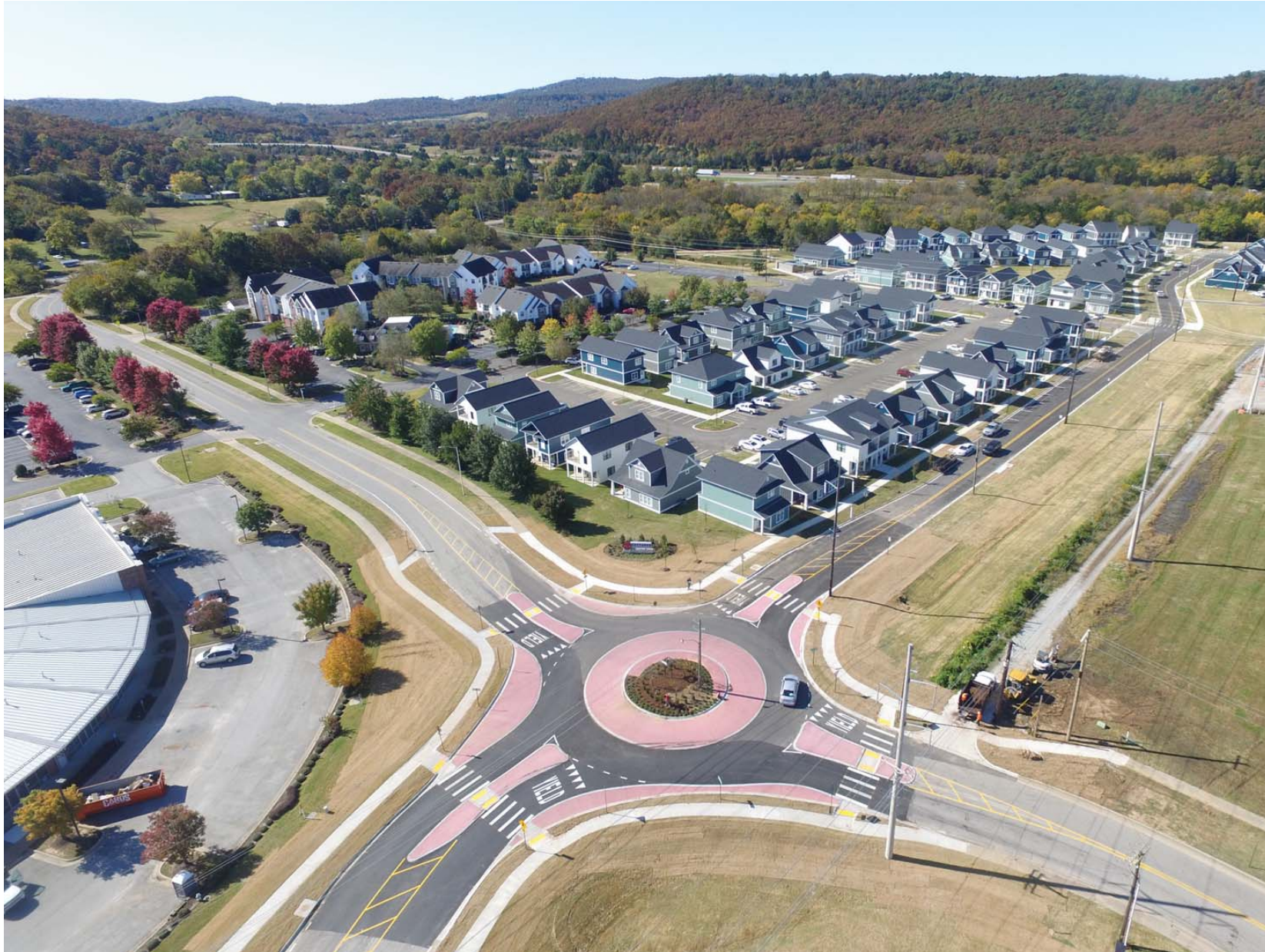
Fayetteville, AR 15th + Beechwood Intersection Improvement
